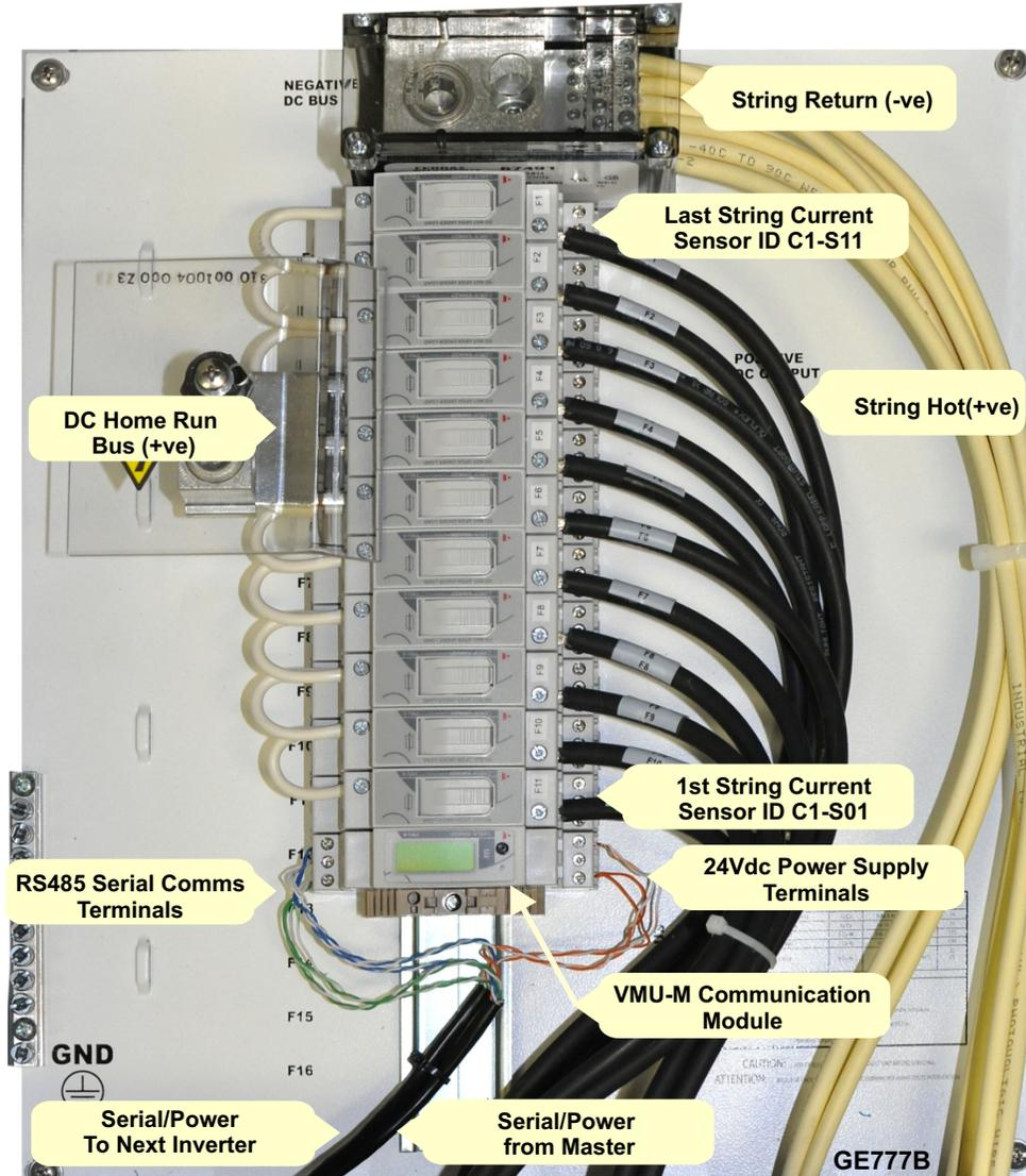
Fig 4 Smart combiner communication wiring using CG VMU-M communications module
